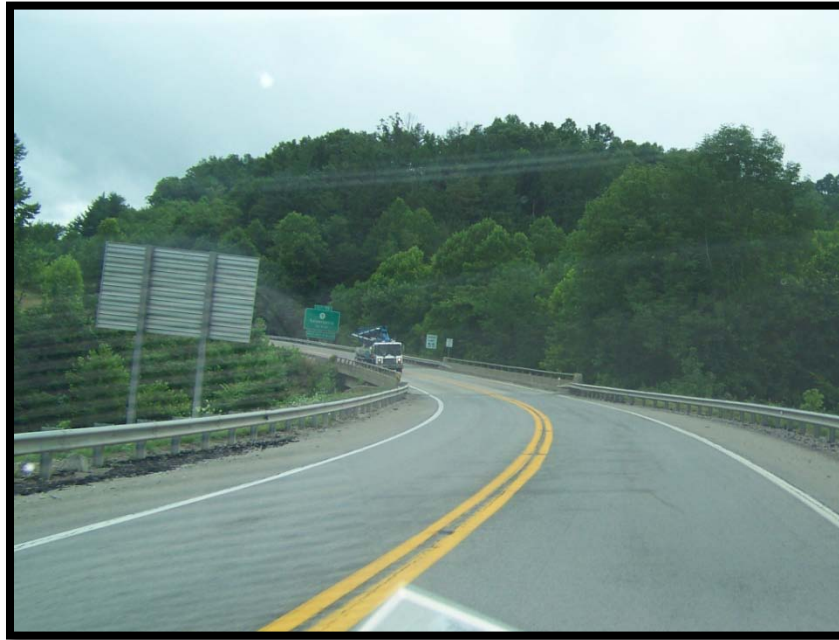
Figure 5: Bridge over Burning Fork
